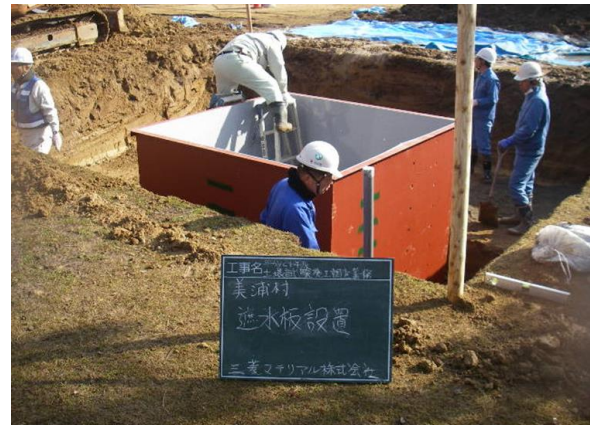
Fig. 1 A trench with an area of 6 m × 6 m and a water impermeable steel frame installed at site A in Miho, Ibaraki prefecture.
