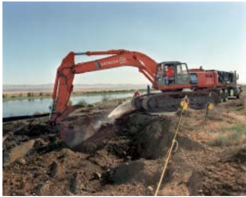
Fig. 18 Hanford Site contaminated soil excavation
