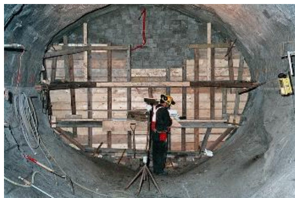
Fig. 5 Photograph Showing the Completed Construction of the Clay Plug
