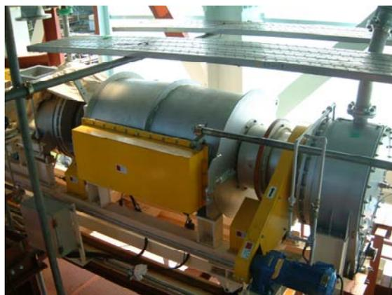
Fig.6 Incinerator for relatively high-level flammable and less-flammable wastes and spent resin.
