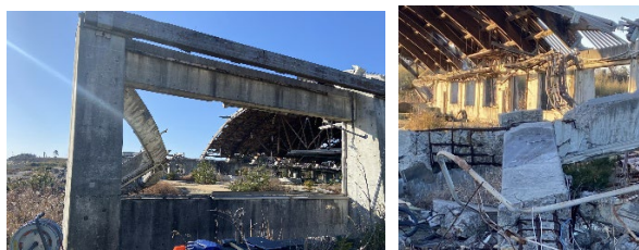
Fig.2 The standing column (the left column in left photo) and the collapsed column (the center column in right photo) surveyed.
