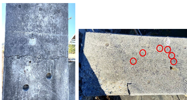
Fig.3 Surface textures of columns surveyed. A large horizontal crack in the standing column (left) and a small crack in the collapsed column (right). Red circles indicate the location of sampling.
